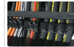
Tank chain cable tubing All cable tubing inside the tank chain uses special made fixtures to avoid cable tangle and rubbing damage.
