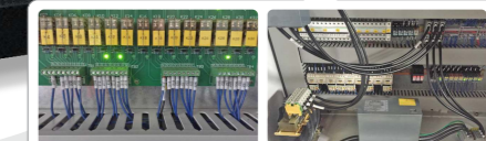
Use Germany IGUS cable and wire, Phoenix terminals, Schneider contactor, the whole machine's wire arrangement is according to European CE standard.
